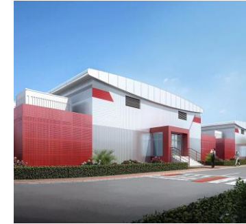
CN04 Location: Greater Beijing Area IT capacity in service: 28MW
