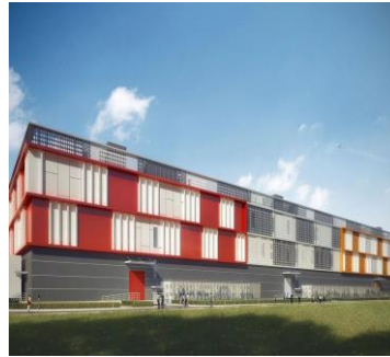
CN06 Location: Greater Beijing Area IT capacity in service: 30MW
