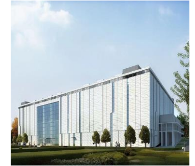
CN05 Location: Greater Beijing Area IT capacity in service: 23MW
