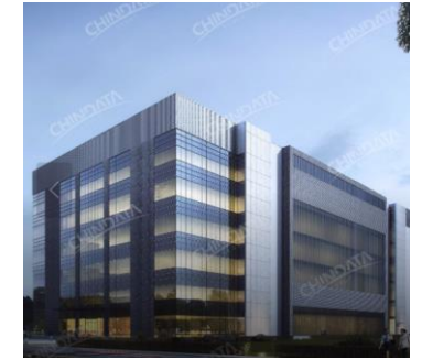
BBY01 Location: Mumbai IT capacity in service: 20MW
