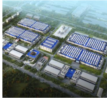
CN01 Location: Greater Beijing Area IT capacity in service: 36MW
