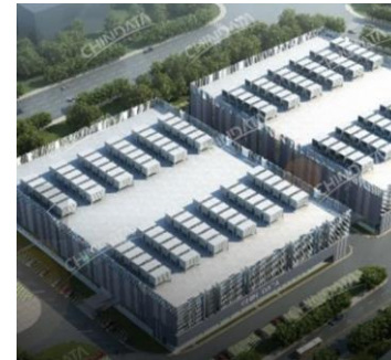
CE01 Location: Yangtze River Delta Area IT capacity in service: 18MW
