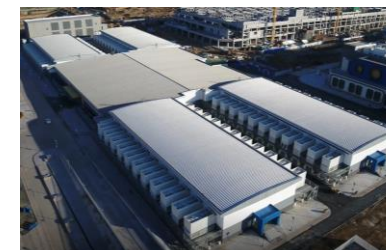
CN14 Location: Greater Beijing Area IT capacity in service: 18MW
